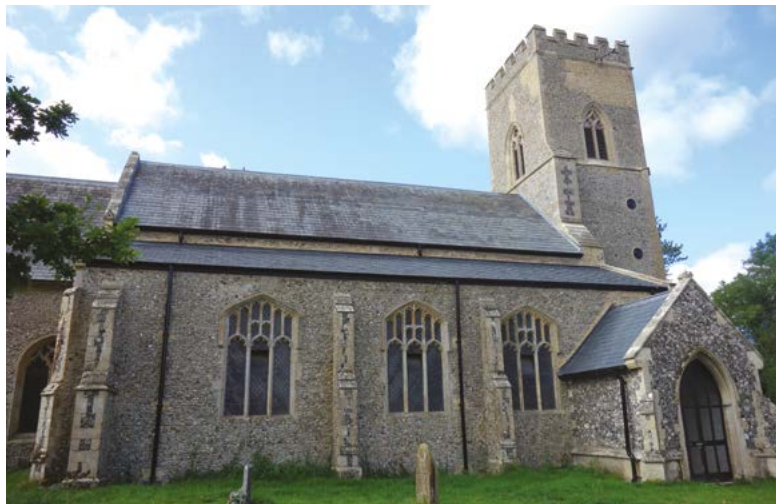
Figure 5: North aisle and porch after 2019 repairs
