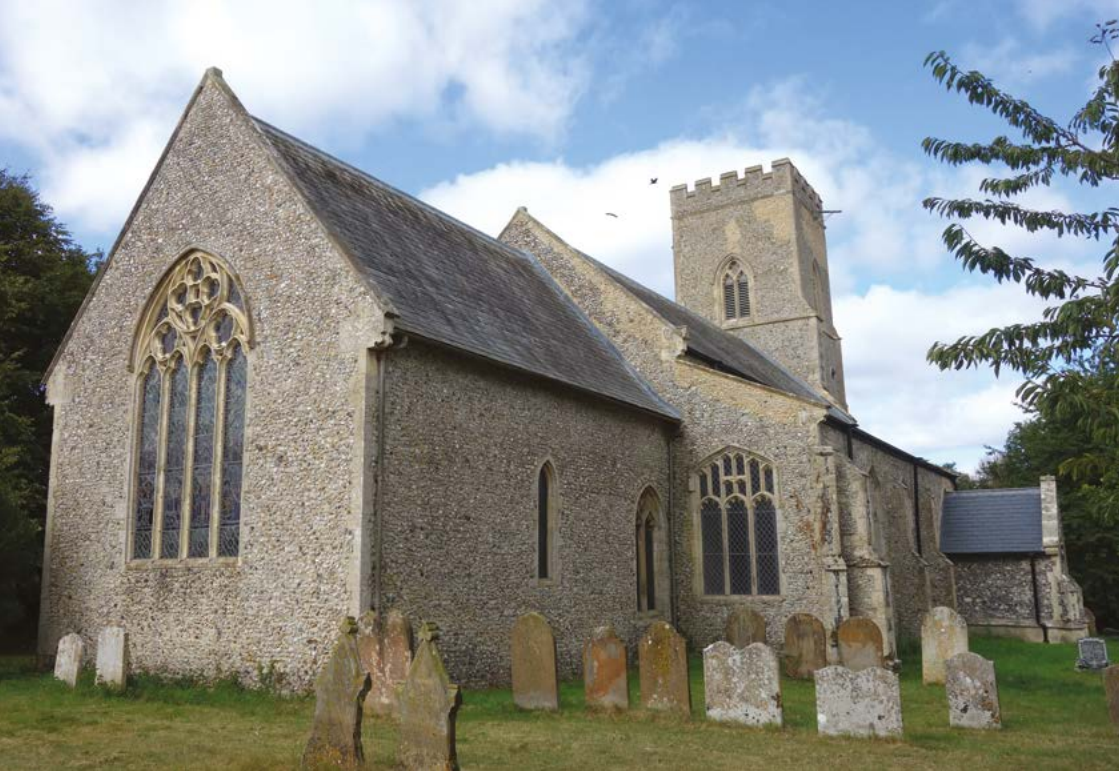
Figure 3: View from the north east
