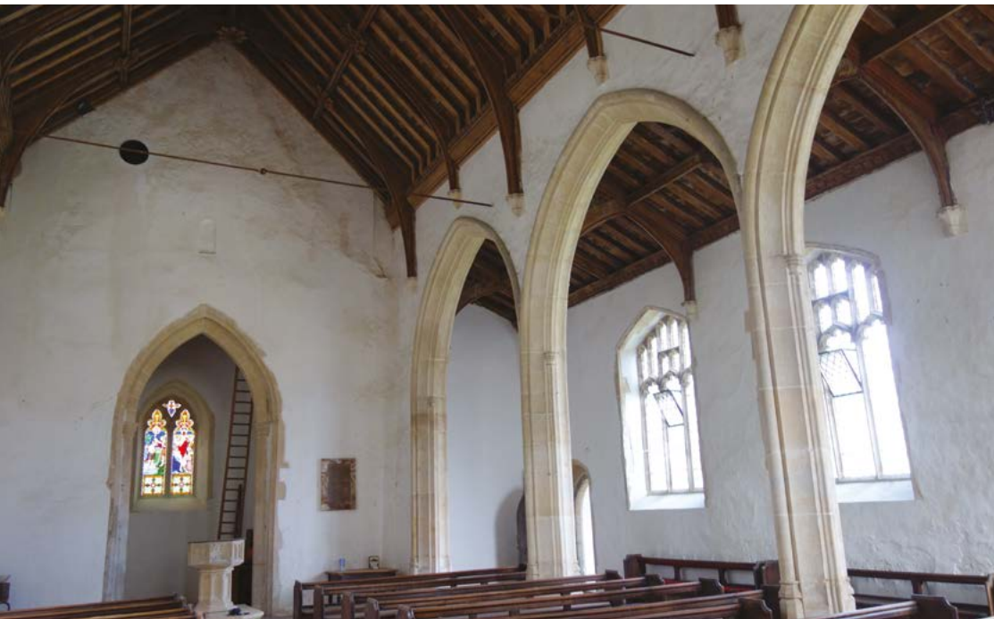
Figure 10: Interior to west
