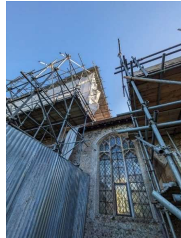
Scaffolding at Wilby, All Saints
