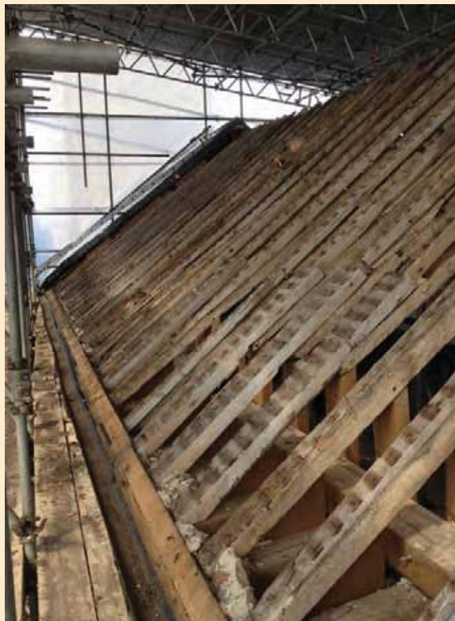
St Michael, Hockering: chancel roof (photo: Nicholas Warns Architects).
